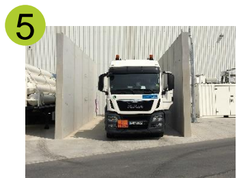
5 Hydrogen filling station
